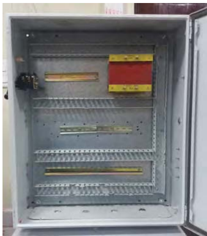
CONTROL PANEL WITH RACEWAYS/DIN RAILS
