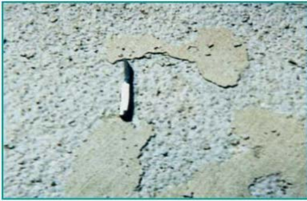
Scaled concrete surface resulting from lack of air entrainment, use of deicers, and poor finishing and curing practices
