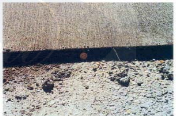
Plasticized, flowing concrete is easily placed in thin sections such as this bonded overlay that is not much thicker than 1 1/2 diameters of a quarter.
